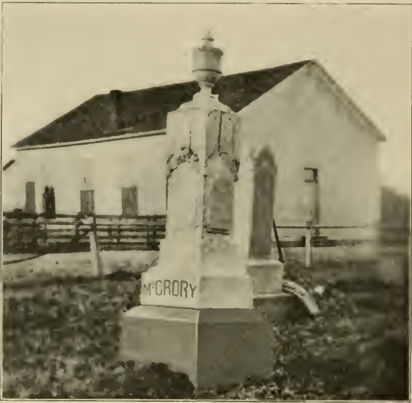
OLD SECEDER CHURCH, NEW CALIFORNIA. (Erected 1852.)
